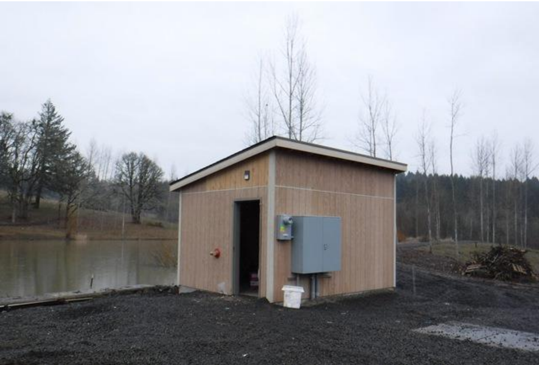
R36301 FIRE PUMP SHED 03.06.19
