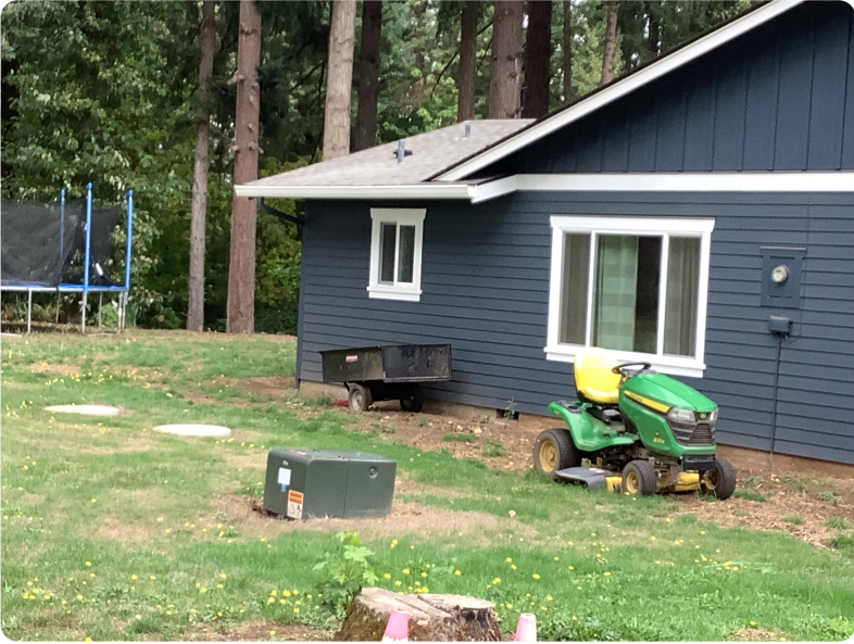
Addition @ 100%. (Back section of House)
