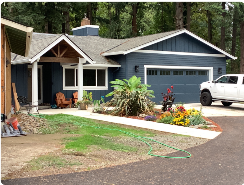
New Attached garage @ 100%.
