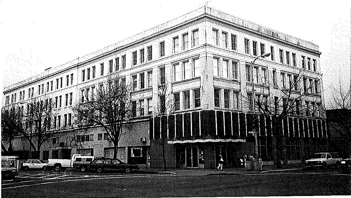
Photograph 3. The Senator Hotel (southwest corner).
