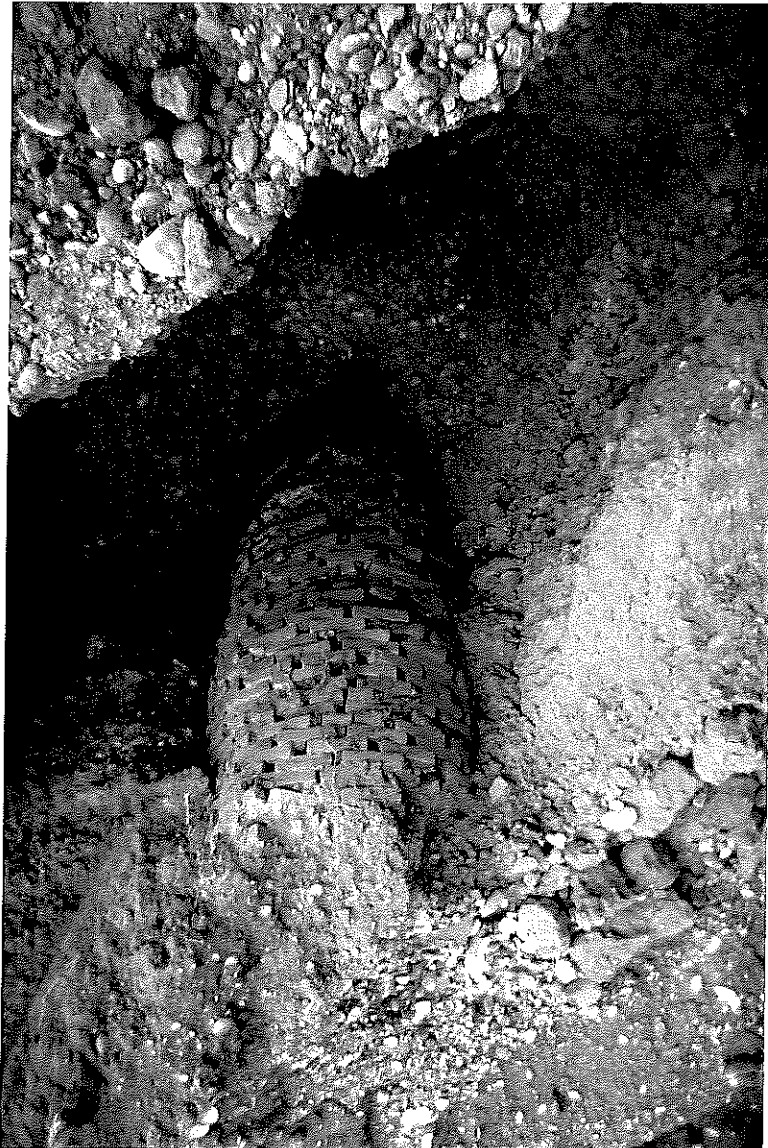
Photograph 6. Site 8 - excavation along dry well.
